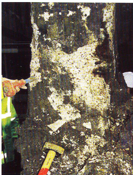
Sulfate attack of 30-year-old bridge sub-structure
