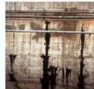
Concrete Cracking With Grease Leakage
