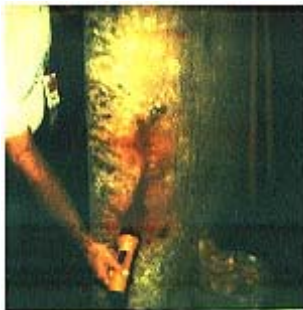
Water Intake Structure Rebar Corrosion
