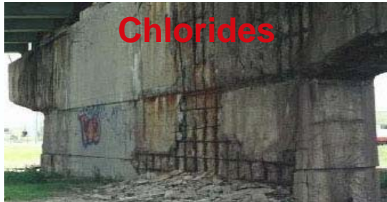
Corrosion of steel reinforcement in bridge superstructure
